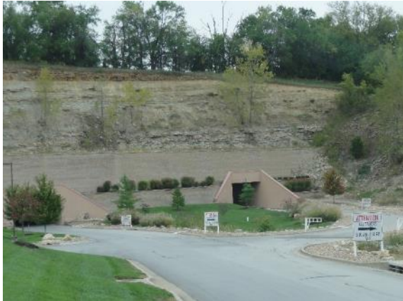
Figure 10. Entrance to the Meritex mined space reuse in Lenexa, Kansas (photo: R. Sterling)
