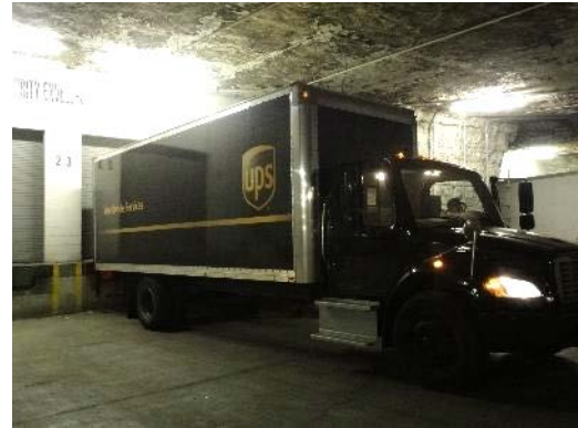
Figure 13. High quality access - Loading dock within the Meritex Lenexa mined space (photo: R. Sterling)
