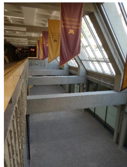
Figure 17. Angled glazing providing light and view to the -2 level at Williamson Hall (photo: R. Sterling)
