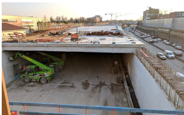
Figure 2. Building a Highway lid (A7 Stellingen, Hamburg, Germany)
