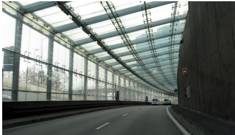
Figure 8. Glazed portal section of Petueltunnel, Munich, Germany
