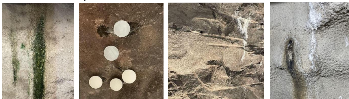
Organic reaction, water collection cups, marks left by drilling tools, efflorescence phenomenon, Formula Center leisure center, personal photographs, november 2023, Helsinki.
