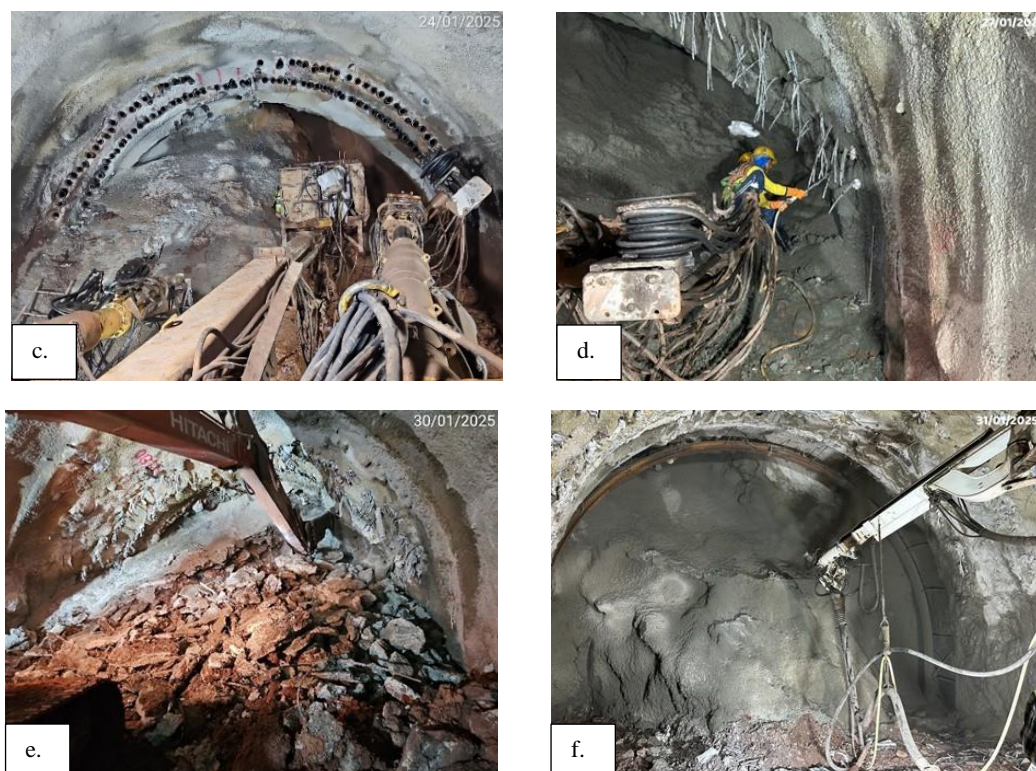
Figure 7. Show the incident roof collapse at STA 0+770.278 (Up track)
