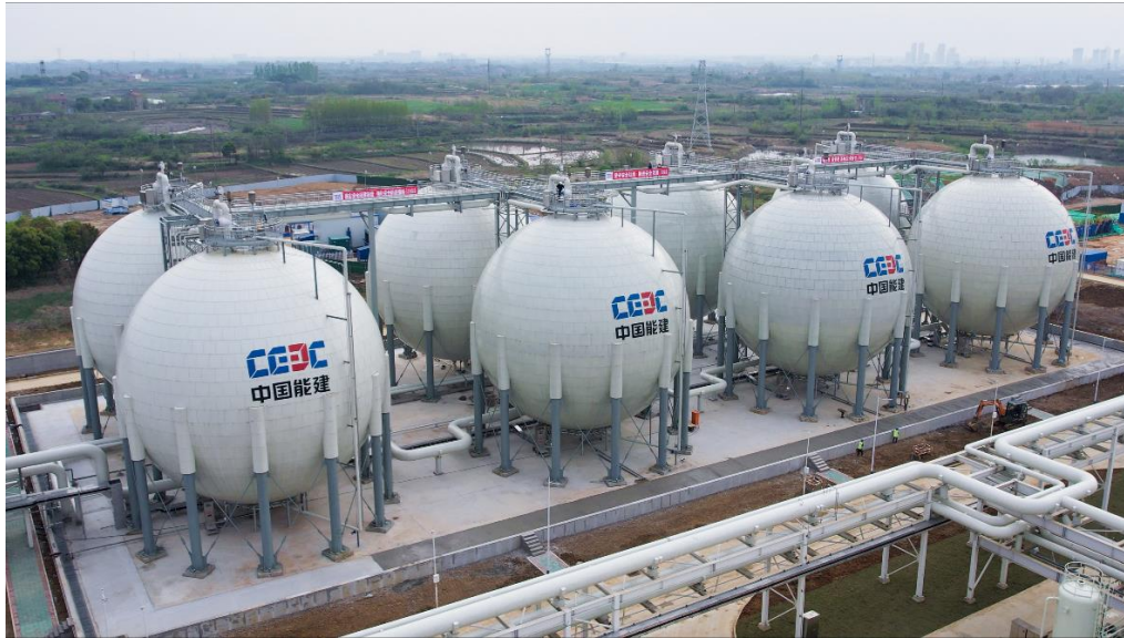
Figure 3. Surface pressure-bearing spherical tanks at the "Nengchu-1" facilities (source: http://en.ceec.net.cn/art/2025/1/10/art_138_2510992.html 24/06/2025)
