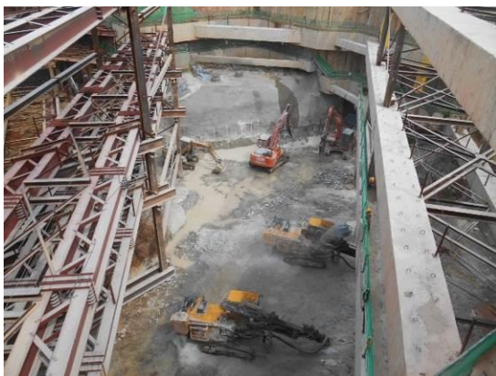
Figure 6. Rock Splitting Method
