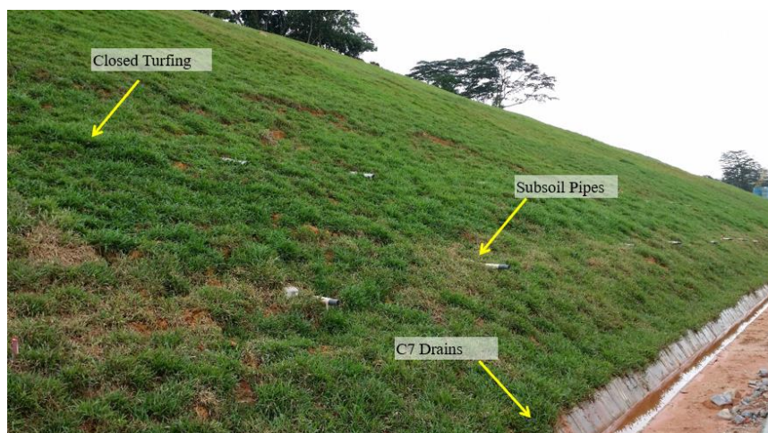
Figure 7. Soil Slopes Surface Protection using turfing, subsoil pipes and cut-off drains
